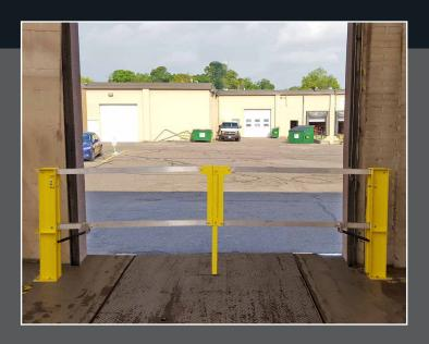
Industrial and commercial facilities often leave their loading dock doors open in the summer for ventilation or in preparation for truck arrival or departure. This open space can cause significant risk for injury and is subject to OSHA regulations 29 CFR 1910.28(b) and 1910.29(b) requiring fall protection measures if the fall to a lower level is 4 feet or greater.
