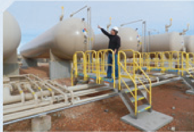
30" vertical clearance, 9' span over pipes.
