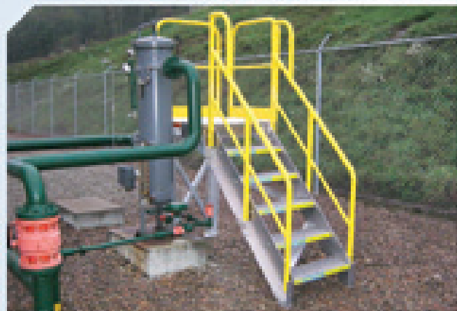
Configure handrail placement for access as required.
