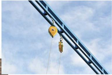
The monorail fall protection system's enclosed track design keeps the tether track trolleys easily rolling so users have free range of motion throughout their work activities. Their tie-off point remains overhead.
